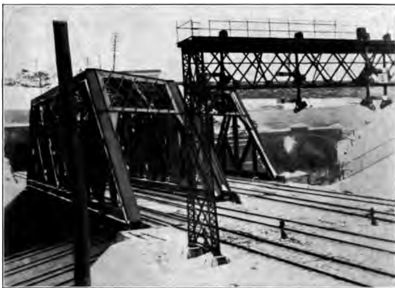
THE BUSIEST TUNNEL POINT IN THE WORLD — AT THE WEST PORTALS OF THE BERGEN TUNNELS, SIX ERIE TRACKS BELOW, FOUR LACKAWANNA ABOVE
